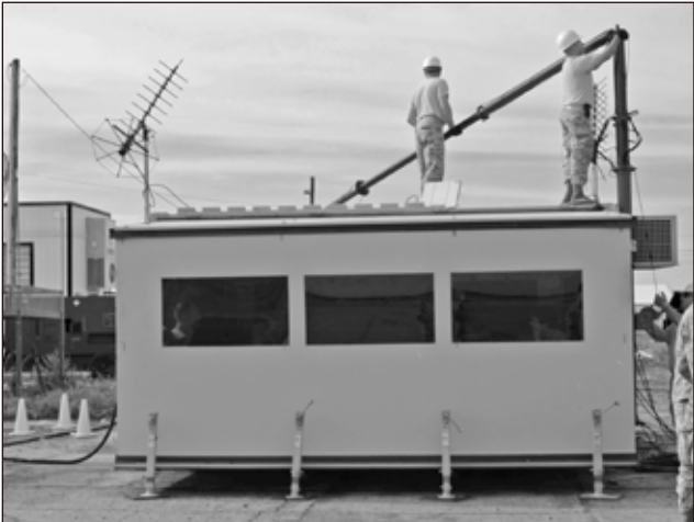
RADIO REPAIR >> Airlift control flight Airmen repair the 50-foot antenna mast damaged by high winds in Colorado at the beginning of Patriot Express.
