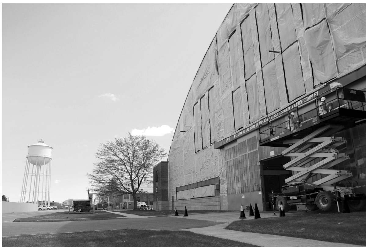
HANGAR FACELIFT Crews replace the front of Hangar 9 April 28. Renovations will continue on each hangar through this summer. The hangars, built in 1940 for maintenance of World War II bombers and fighters, now house offices and equipment. (photo by Master Sgt. Andrew Biscoe)
