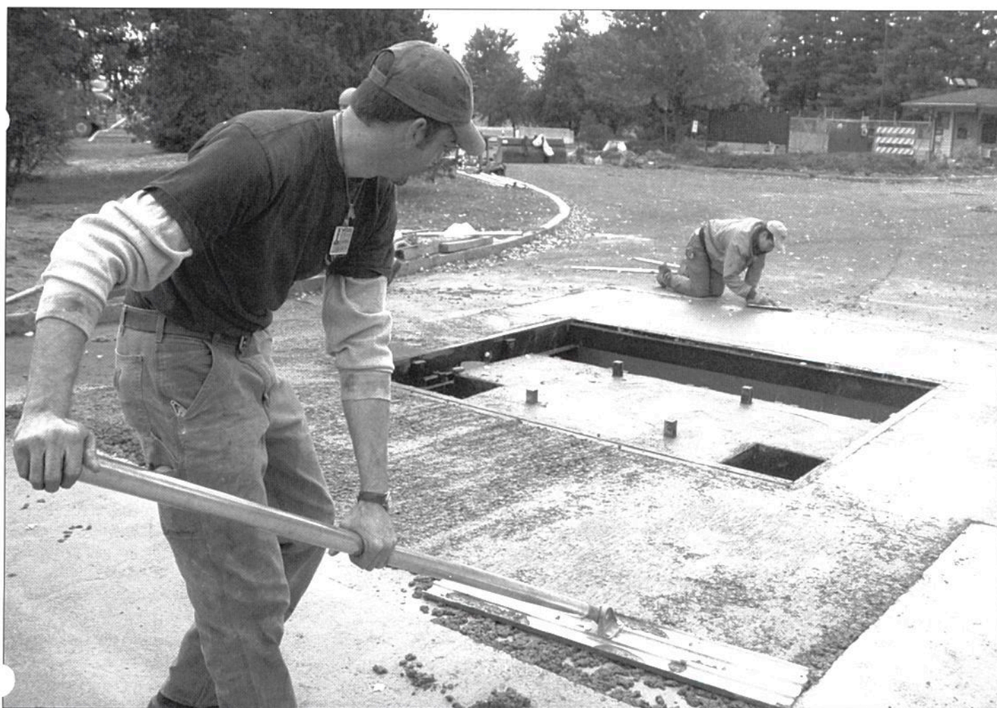
SMOOTH SURFACING >> Clayton Gray, with Secure Applications Inc., smooths out concrete over one of the pop-up barriers at the James Street Gate. The barriers are part of new security measures taken to protect Westover. Crews have installed the barriers at the new Westover Road gate as well.
