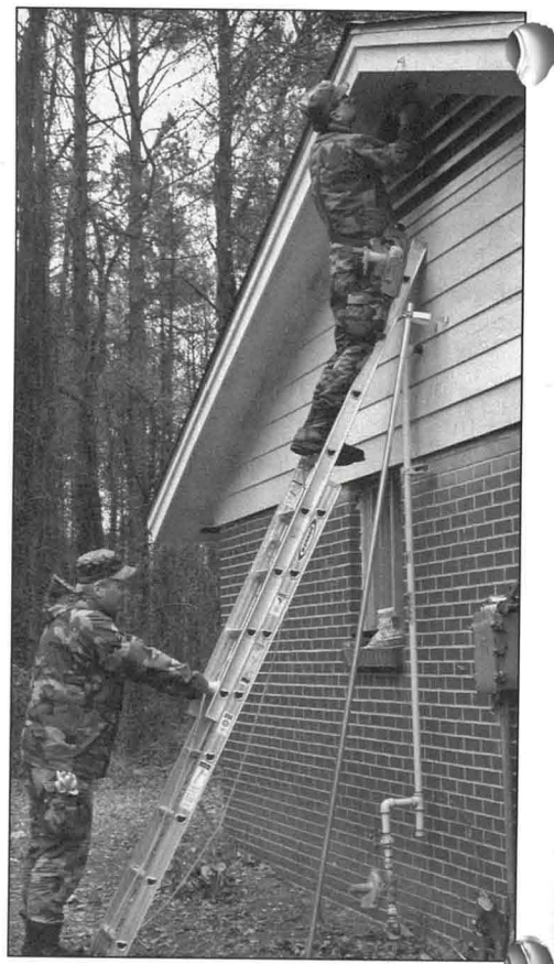
WIRED — SrA. Keith Davis holds the ladder while TSgt. Robert Brown installs a wiring bracket for a fire alarm system while renovating buildings for the new CE school.
