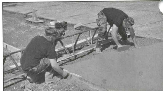
ROAD TO READINESS — From tar to concrete, Westover civil engineers paved the way to a successful annual tour at RAF Lakenheath in England in April and May. At left, SMSgt. Dean Pursell drives the paver as (l. to r.) SSgts. Russell Huther and Joshua Hebert and TSgts. Kenneth Crawford and Warren Coleman provide assistance. Above, Pursell and Hebert screed concrete to smooth the surface.
