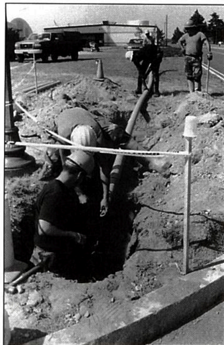
IN THE LINE OF DUTY -- Members of the 838th Engineering Installation Squadron at Kelly AFB, Texas install miles of conduit, innerduct and cable to prepare Westover for changeover to fiber optics. In above photo, workers bore a hole under the roadway, and below, workers feed conduit underground through manhole system.
