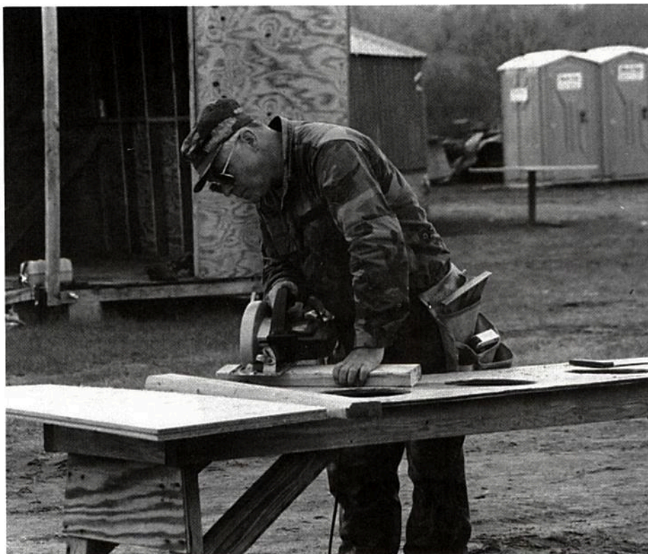
SAW DOCTOR — SSgt. Douglas Cowan, 439th CE structural journeyman, trims a 2" x 4" beam for a perfect fit.
