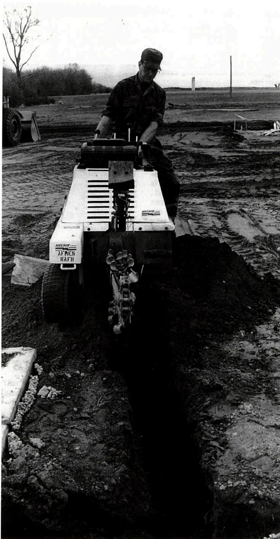
EXCAVATOR — MSgt. Joseph Voutour, 439th CE electrician, uses a trenching machine to cut a trench to lay conduit lines.
