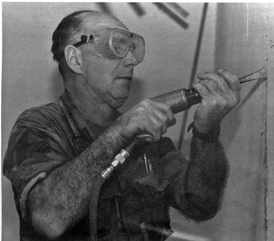
POWER CHISELING -- SMSgt. James Devitt, electrical superintendent, cuts a new doorway in a masonry wall while refurbishing maintenance offices.
