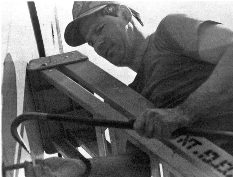
PRYING HIGH -- MSgt. John Mailo, a structural technician with the 439th CES, removes a steel plate from a baffle at the U.S. military firing range.
