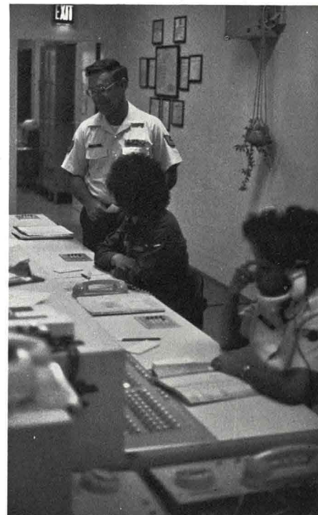
MSgt. Harold Crapo, A1C. Stacia Hicks and Amn. Patti-Jo Stallworth work the Rhein-Main base administrative switchboard.
