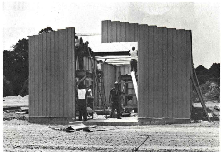
Acid Chemical Storage Building
