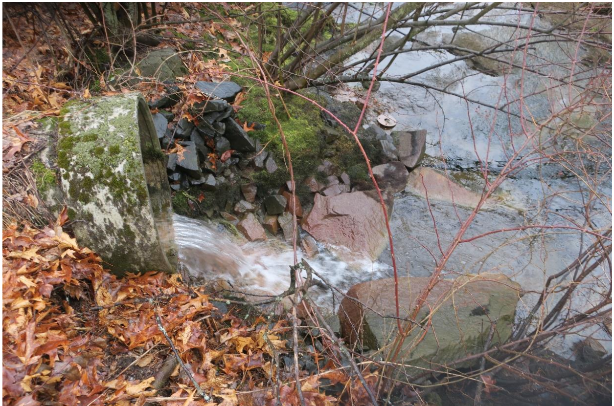
Photograph 4 - Outfall 002 oil/water separator discharge pipe
