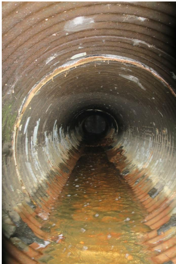
Photograph 6 - Outfall 003 discharge pipe showing disconnected joints and corroded flowline
