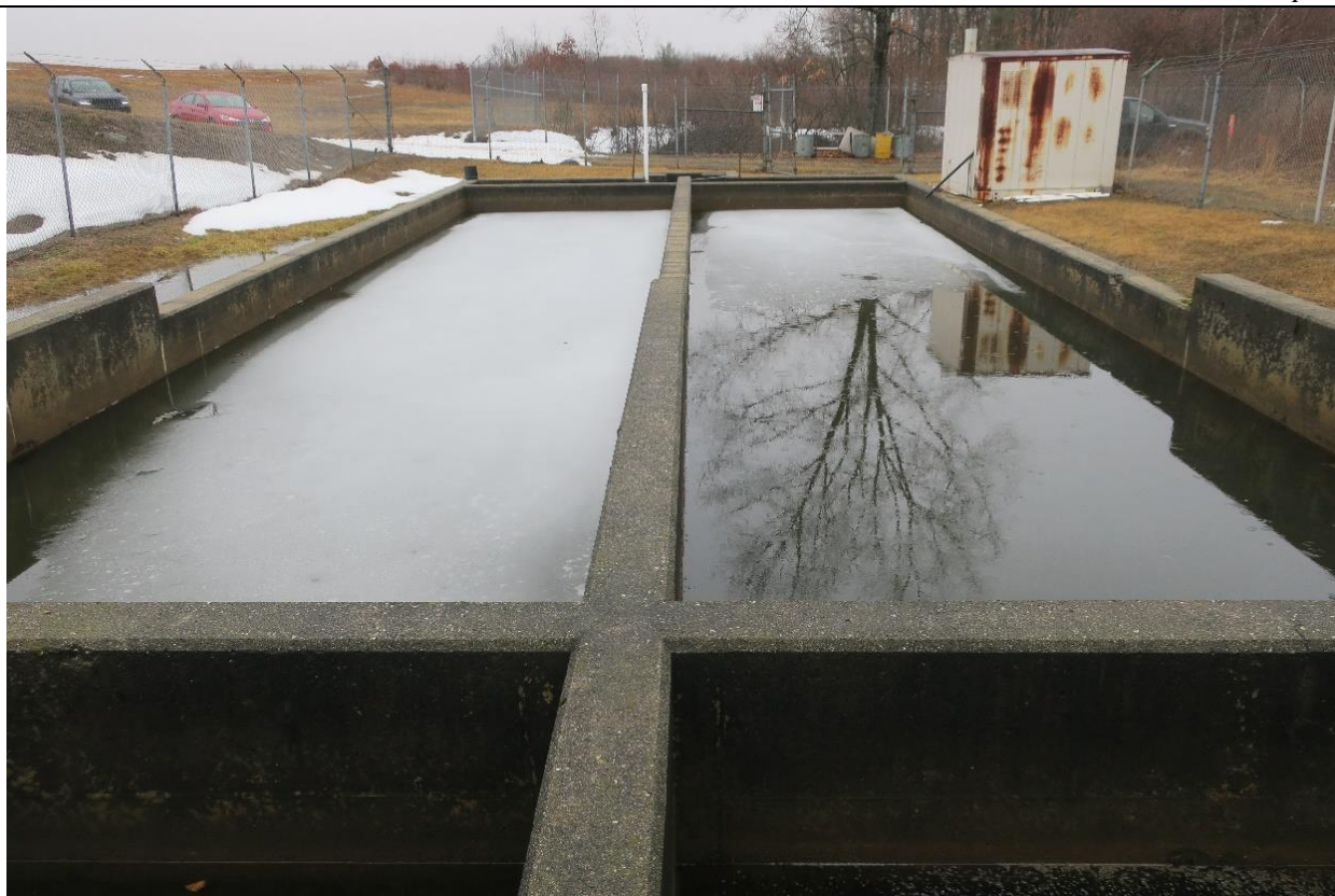
Photograph 1 - Outfall 001 oil/water separator
