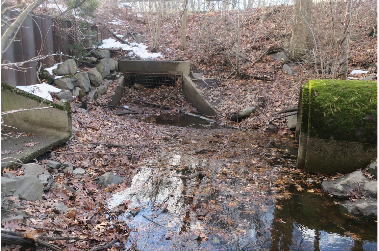
Photograph 7 - Outfall 004, debris buildup on security grate covering culvert
