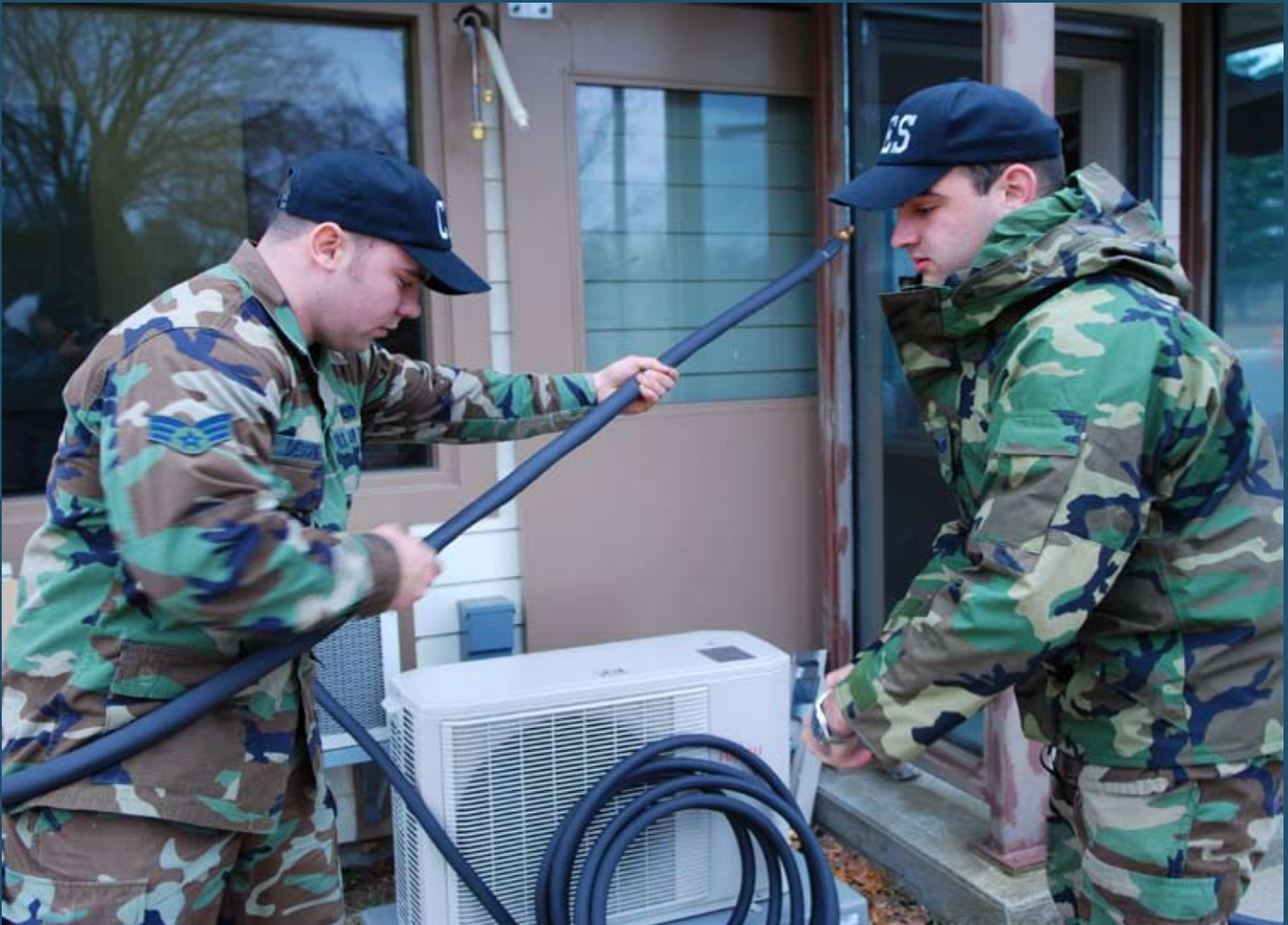
SKILLED LEVEL >> Senior Airman Garret H. Deschenes, 439th Civil Engineering Squadron, left, and Senior Airman Matthew D. Savard, work on a ventilation system by the James Street gate during 3-level training on the April A UTA. The Airmen were part of an on-the-job work order coordination program between the base civil engineer and CES. It is an ongoing training enhancement program designed to help more quickly qualify reserve enlisted engineering Air Force Specialty Codes. (photo by Senior Airman Michael Lanza)
